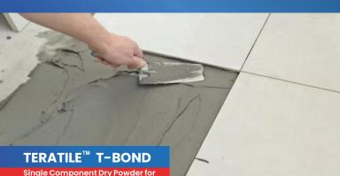
**Cement based Slurry**
