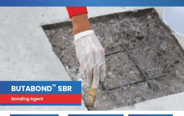
For joint new and old slab, RCC repairing works, injection grouting.
