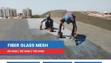
After applying first layer of waterproofing as per the requirements by using appropriate equipment. Lying of the net over the first coat of the application done, positioning it in the vertical or horizontal directions and overlapping the joints by at least 10 cm.
